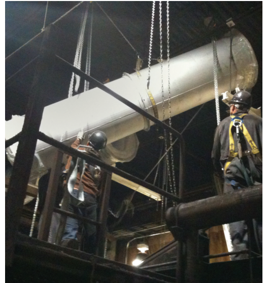
Installation of High Heat Ducting
