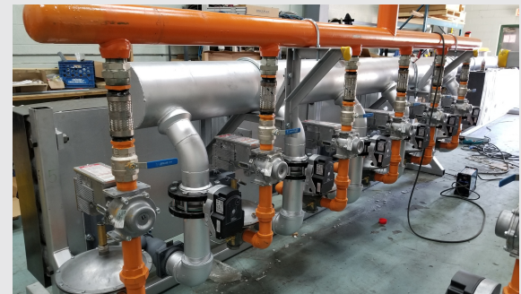
Manufacturing of modular burner and fuel train system
