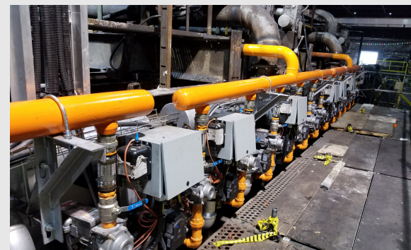
Installation of new burner system on the original furnace
